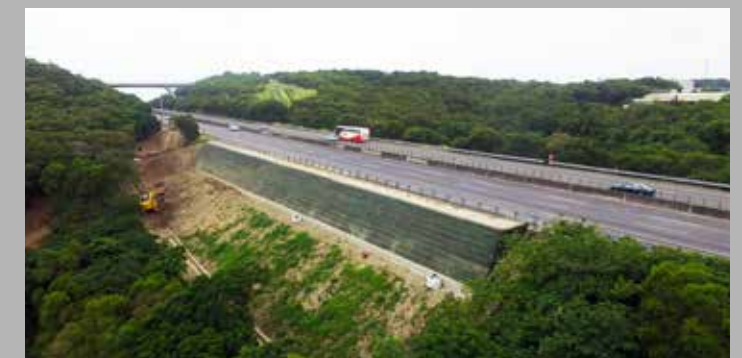
4. Embankment and Abutment Construction
