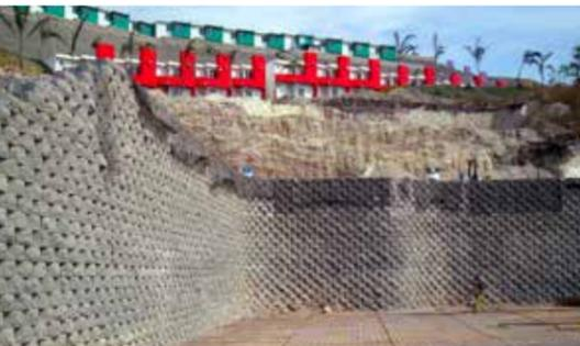
The ACEGrid® MSE wall allowed engineers to integrate cut, fill, and retaining structure into one step which made the site preparation much straightforward. Compacted fill reinforced with ACEGrid® satisfied both static and dynamic loads and therefore becoming a perfect seismic-stable structure. For aesthetic requirements, the designer specifically selected modular concrete blocks as the face of the MSE wall to match well with the appearance of the surrounding housing complex.
