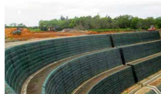
The mechanically stabilized earth construction method is used to complete the reinforced earth retaining wall at a height of 29 meters and the slope top drainage system.
