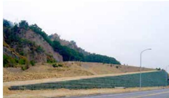
The stiffened earth embankment is used as the main structure for earth and stone treatment as it blocks and guides the earth and stones into the temporary accumulation area. A dredging channel is setup at the top of the embankment in order to transport and accumulate earth and rocks for reuse.
