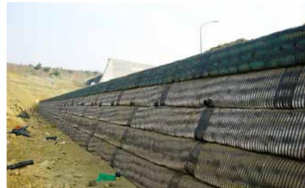
Fig.1 Laying of the Geotextile on the Inside of the Reinforced Earth Embankment
