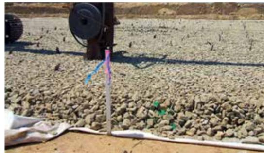
When the Prefabricated Vertical Drains (PVDs) are used along with the ACETex® PET geotextiles, the PVDs can accelerate the excess pore water dissipation in the soil, while the ACETex® PET have separation and reinforcement effects. This can increase the soil shear strength, reduce the amount of compression, and increase the bearing capacity upon completion of the construction work.
