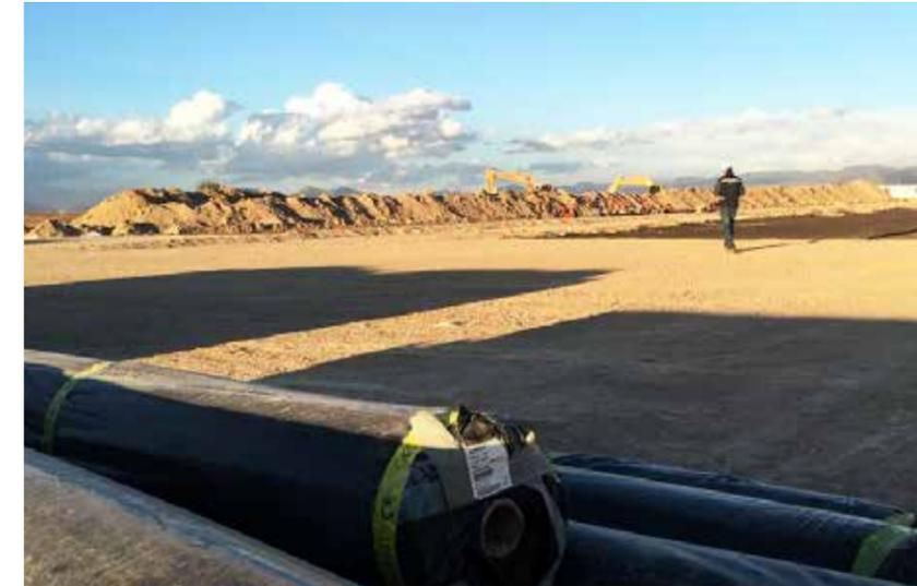
ACETex® geotextiles and ACEGrid® geogrids are used together, as the former separates the weak strata, while the latter reinforces and stabilizes the strata. ACETex® geotextiles and ACEGrid® geogrids can jointly disperse the building load and avoid soil subsidence to stabilize the strata.
