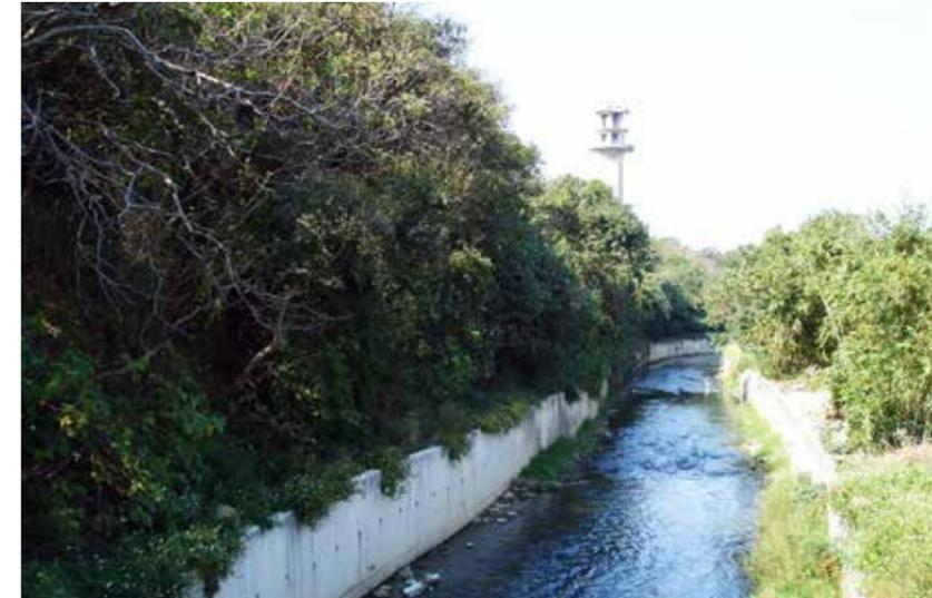
A 10m high-strength earth-retaining wall with a total length of more than 250m was built, and the top of the reinforced earth structure was used as a 15m-wide composite contact road.
