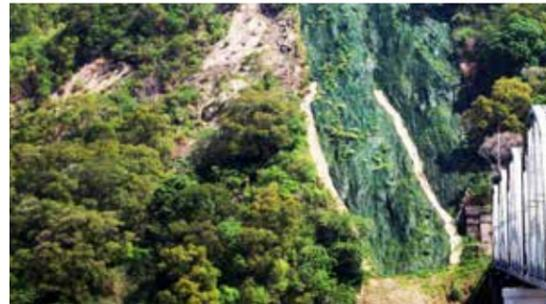
The three-dimensional ACEMat™ R with diamond-shaped wire mesh composite was used to replace the traditional concrete slope which induces significant loading on the slope. Also, soil nail is used along the fractured zone to stabilize the slope surface, control the erosion of the collapsed ground and facilitate re-vegetation.
