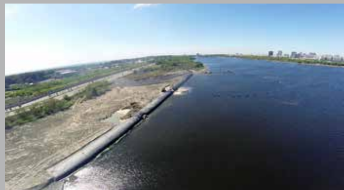
3. Seawalls and Bulkheads
