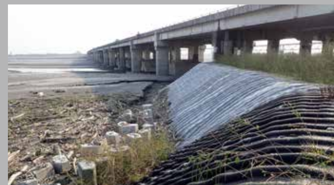
6. Pier Scour Protection
