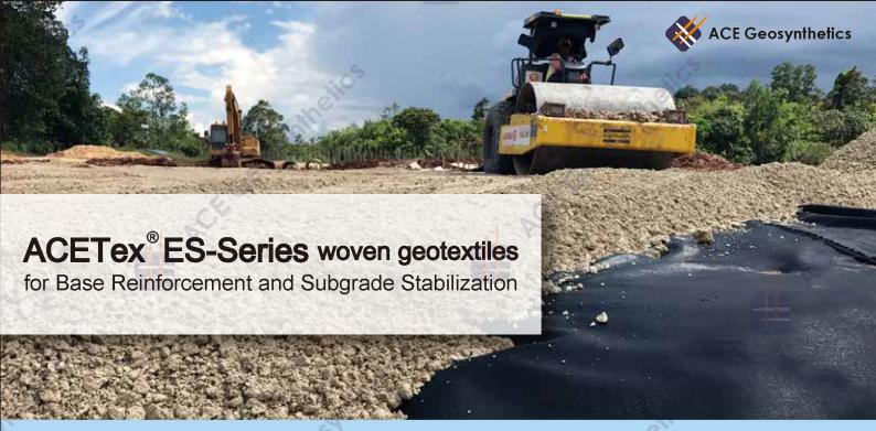
ACETex<sup>®</sup> ES-Series woven geotextiles, fabricated with self-developed high tenacity polypropylene yarns and well-designed texture, perform exceptionally well in separation, filtration, and reinforcement functions altogether to enhance the safety, reliability and serviceability of paved and unpaved roadways.
